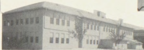
West Side Lenapah H.S. Building, Bus-Loading Entrance
