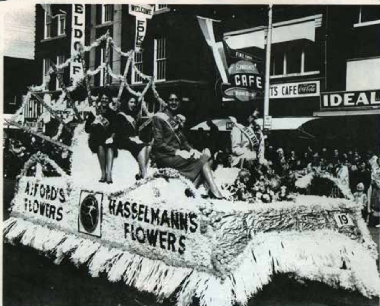
Photo Courtesy of Heartland Cement
