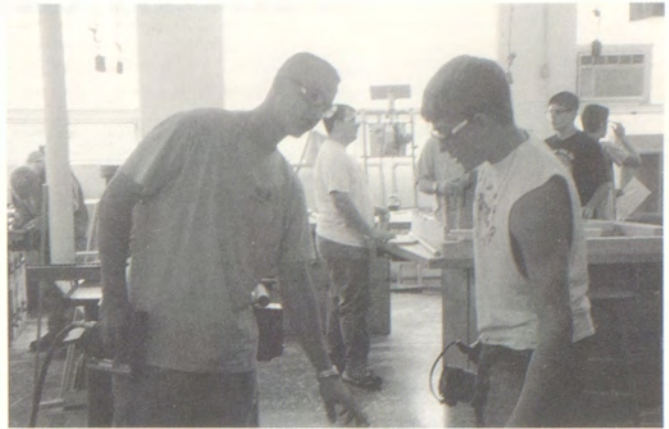
Eddie Swearingen and Dustin Johnson work together to build a cabinet.
