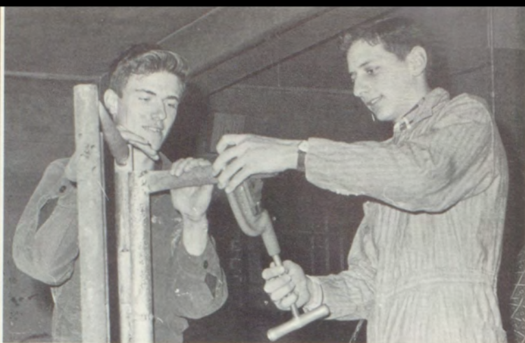
USING A pipe cutter, Gerald Sullivan makes a squeeze chute. Robert Applebaugh lends a helping hand.
