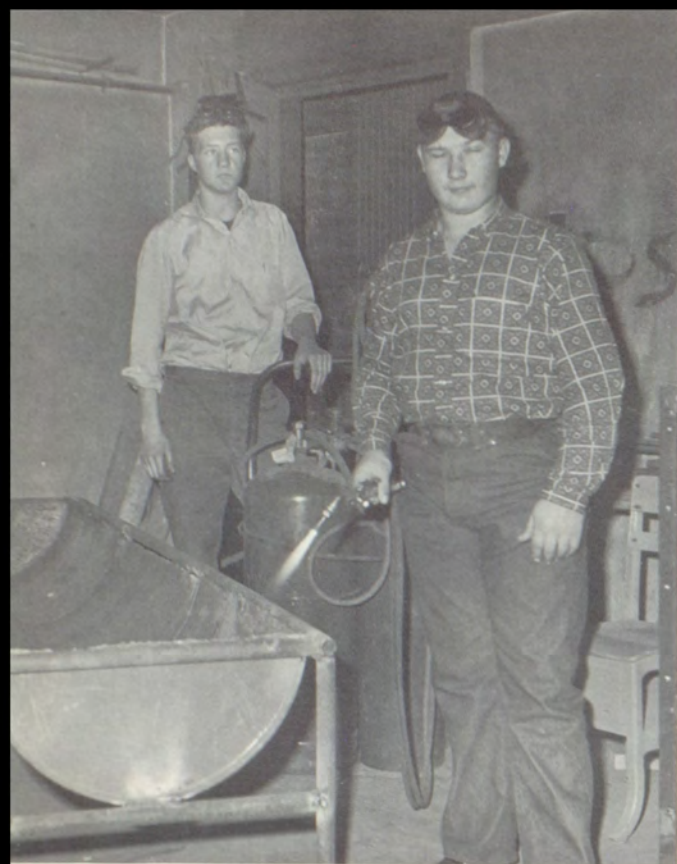
PUTTING THE finishing touches on the feed bunks Tom Zinser uses the acetylene torch with Carl Hilyard at the controls.
