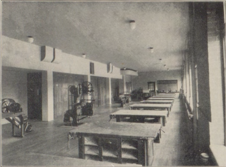
The Woodworking Shop
