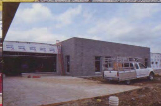
The new administrative offices begins to take shape.
