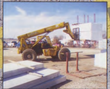
The sight of heavy equipment moving construction materials was commonplace in 2011.
