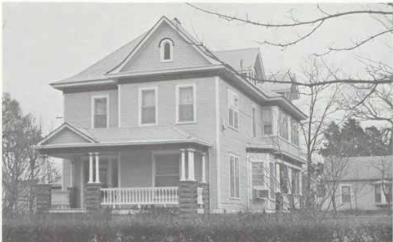
This large home at 118 South Twelfth Street (above) was constructed by J. B. Kunze and Arthur Hurd in 1903 for R. L. "Bob" Scott who was in the grocery business. The house is supported by nine feet of stone foundation, six feet of which is underground and there are matching stone posts by the sidewalks. In 1913 two bedrooms and a sleeping porch were added making a total of eleven rooms in the home. The small, paired and tripled columns with doric capitals and the wide frieze board have been painted to accent the Victorian flavor of the home. The home at 316 South Penn (below) was built about the same time for Curtis Otwell.
