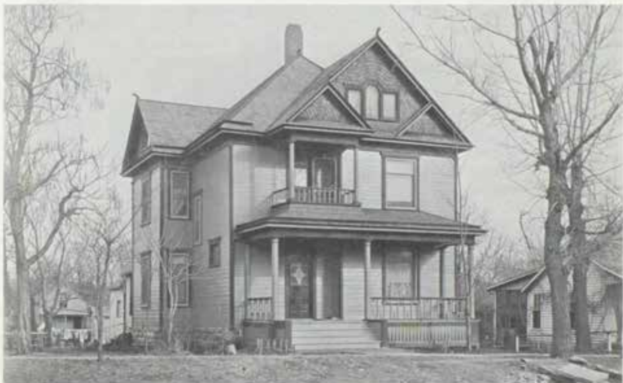
This large home at 118 South Twelfth Street (above) was constructed by J. B. Kunze and Arthur Hurd in 1903 for R. L. "Bob" Scott who was in the grocery business. The house is supported by nine feet of stone foundation, six feet of which is underground and there are matching stone posts by the sidewalks. In 1913 two bedrooms and a sleeping porch were added making a total of eleven rooms in the home. The small, paired and tripled columns with doric capitals and the wide frieze board have been painted to accent the Victorian flavor of the home. The home at 316 South Penn (below) was built about the same time for Curtis Otwell.
